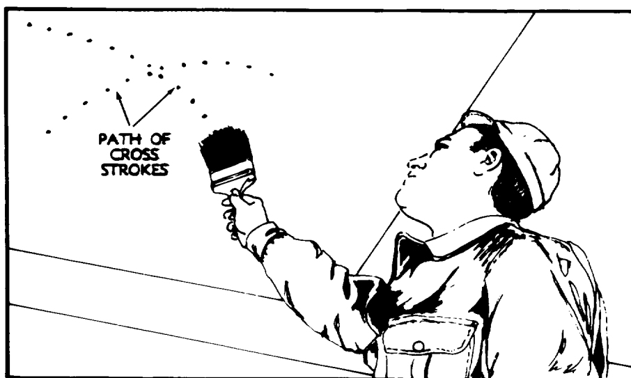
B. TECHNIQUE FOR PAINTING A CEILING.
